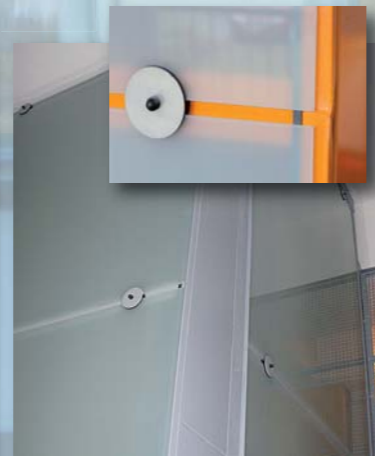
Variant 2 Lining with milky safety glass on discs
