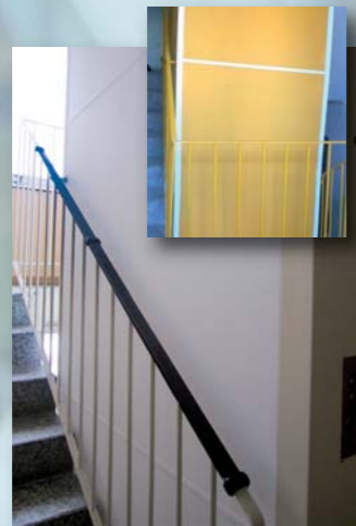
Variant 1 Lining with Rigips boards
